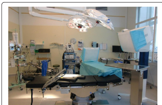
Figure 2 Two MLAF units in an OR. Photo from South Hospital (Södersjukhuset), Stockholm.
